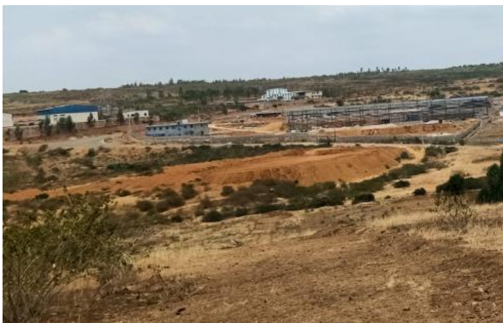
FIGURE 6-4: STOCKPILING OF EXCAVATED SOIL
